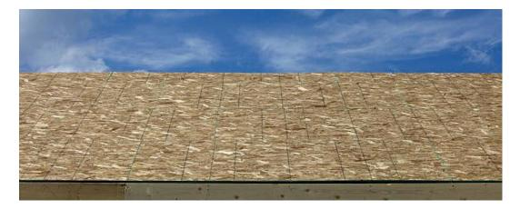
The resins and glues found in OSB products can present a bonding challenge for self-adhered underlayments. There is typically a smooth side and a textured side to the OSB. Carlisle WIP products should be applied directly to the textured side of OSB sheathing for best adhesion. Carlisle WIP Products offers a variety of self-adhering roofing underlayments which include WIP GRIP, WIP 100, WIP 100SG, WIP 250HT, and WIP 300HT.
