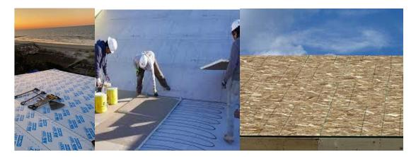
Many non-standard substrates can make proper adhesion of self-adhered roofing underlayments a challenge, such as ISO boards, fire-treated plywood, gypsum products, structural concrete, DensDeck<sup>®</sup>, and even OSB. Fire-treated plywood that contains excessive moisture, inconsistent ingredients in OSB and ISO surfaces, porous concrete, and dust often found on gypsum surfaces can all be bond breakers.
